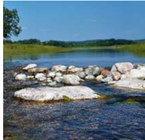
Figure 2.10. Fish Lake dam modification to rock rapids to facilitate fish passage in the Pelican River.
