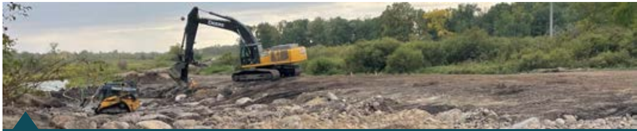
Construction on Rice Lake Wetland Restoration. Credit: PRWD.
